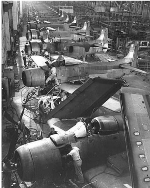
A Douglas Aircraft AD Skyraider production line at El Segundo in 1956 (Photo courtesy of the Boeing Company via Patricia McGinnis)
