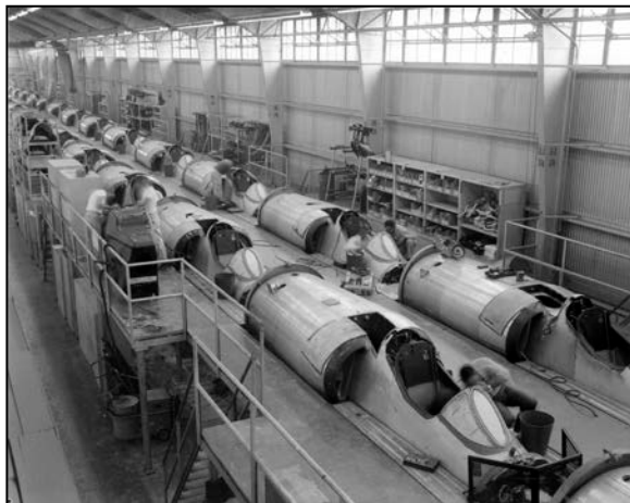
Fuselage assembly at Building 244 in 1959
