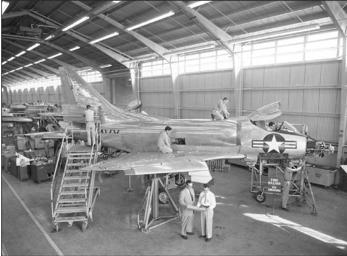
The A4D final assembly line on 3 March 1955. This aircraft assembly building was later converted into the Fitness Center (Building 242) at Los Angeles AFB. The A4D was the only aircraft assembled within the property of Los Angeles AFB. (Photo courtesy of Boeing)
