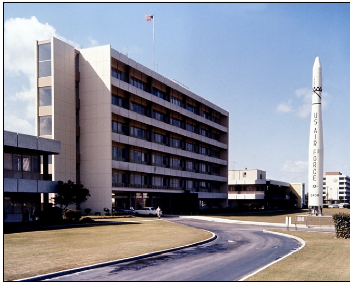
The Building 105 headquarters building and the Thor Agena display in Area A. The Thor Agena stood in front of the building from 1964-1975
