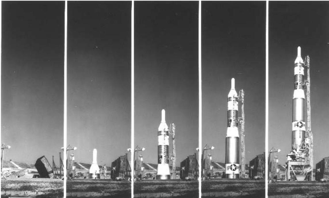
*A Titan I missile emerges from its silo at Vandenberg's Operational System Test Facility in 1960. The Titan I was stored and fueled in a hardened underground silo, but an elevator had to lift it out of the silo before it could be launched. The entire launch sequence took about 15 minutes. Ultimately, the Titan I was deployed in 54 such silo-lift launchers divided among seven operational sites. All became operational in 1962, and all were inactivated in 1965.*
