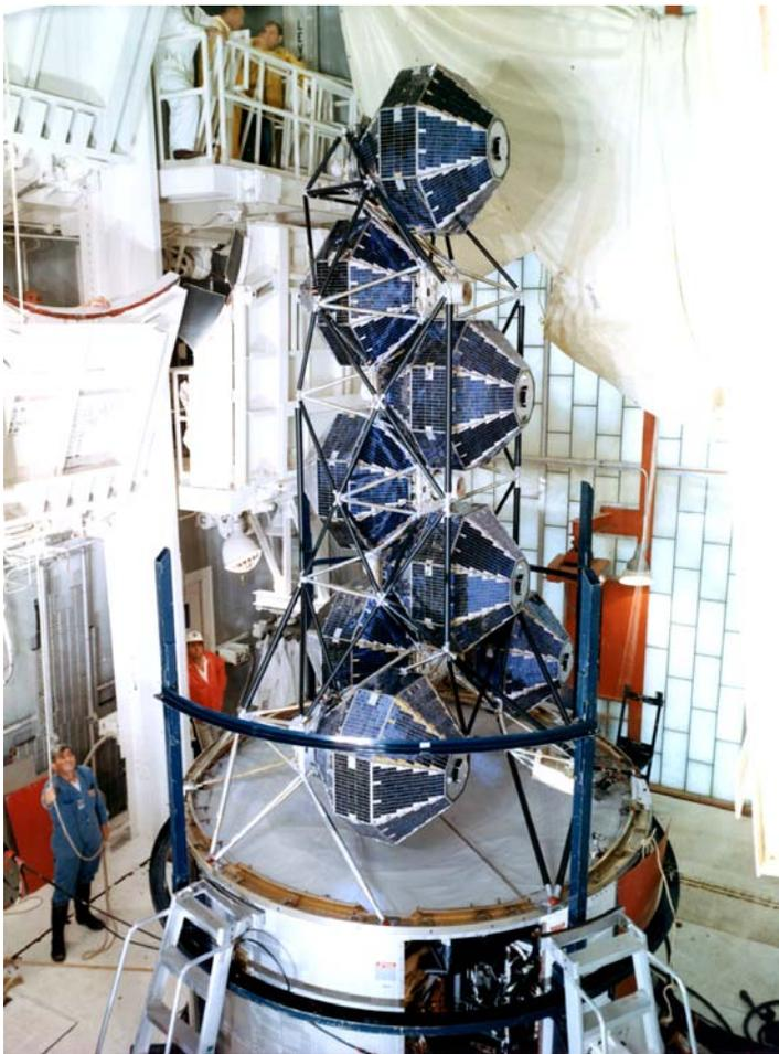
*Left: The payload fairing is being installed on Titan IIIC-16 at Cape Canaveral. Enclosed in a dispensing mechanism are the last eight satellites of the Initial Defense Communications Satellite Program (IDCSP), successfully launched on 13 June 1968. The IDCSP satellites were small and very simple, with no batteries and no active attitude control system. The dispenser ejected them one at a time into a near-synchronous orbit.*
