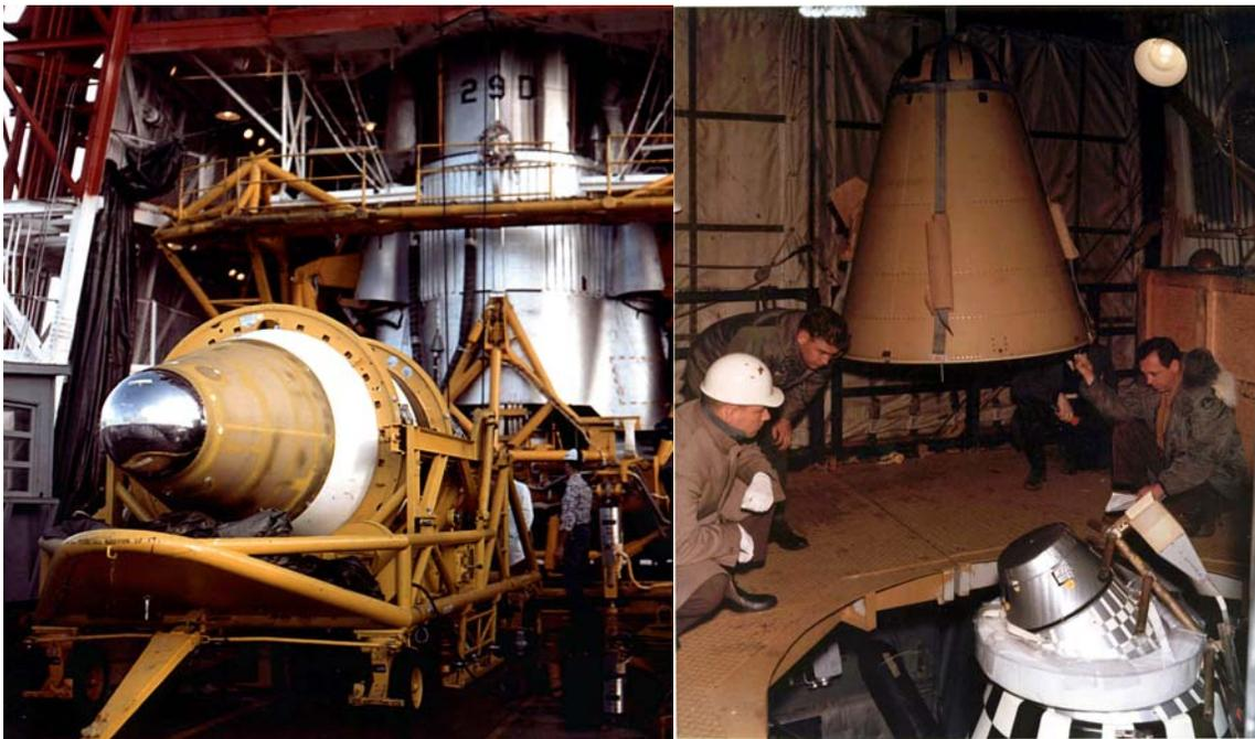
*Left: The Agena spacecraft for MIDAS I waits for installation on Atlas 29D before its unsuccessful launch on 26 February 1960. Right: The payload for an advanced version of MIDAS, known as AFP 461, is covered with the Agena's nose cone before its unsuccessful launch as MIDAS 6 on 17 December 1962.*
